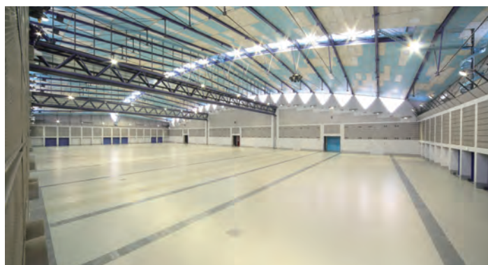
Main Bldg. Exhibition Hall
