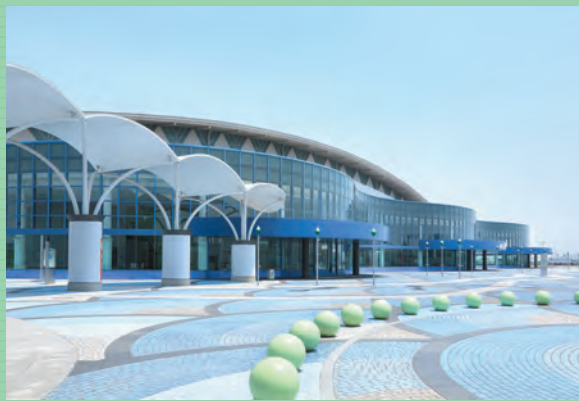
Main Bldg. Exhibition Hall
